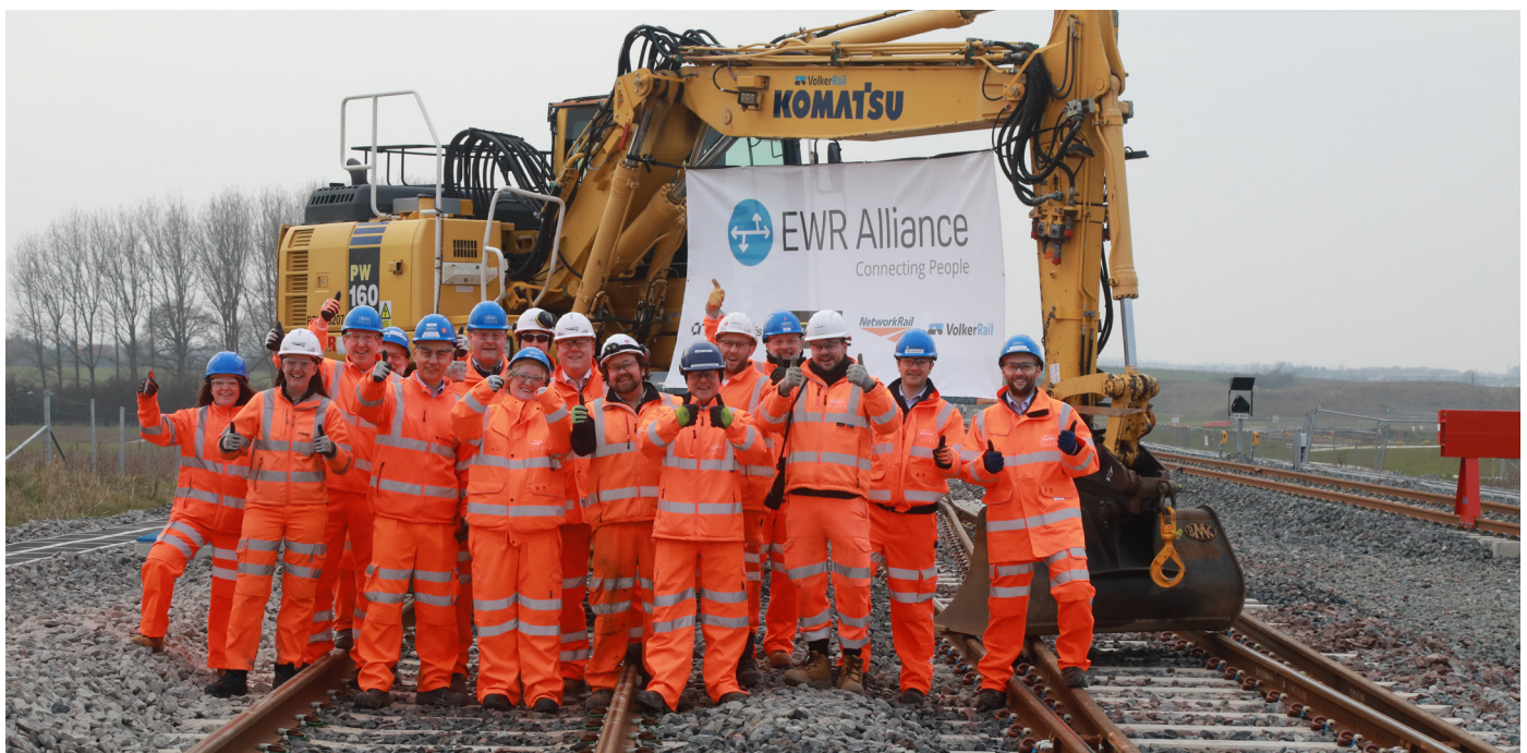
The East West Rail Alliance team marking the completion of track construction from Bicester to Bletchley, March 2024
