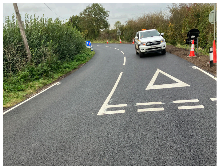
Completed reinstatement works on Herds Hill, October 2023
