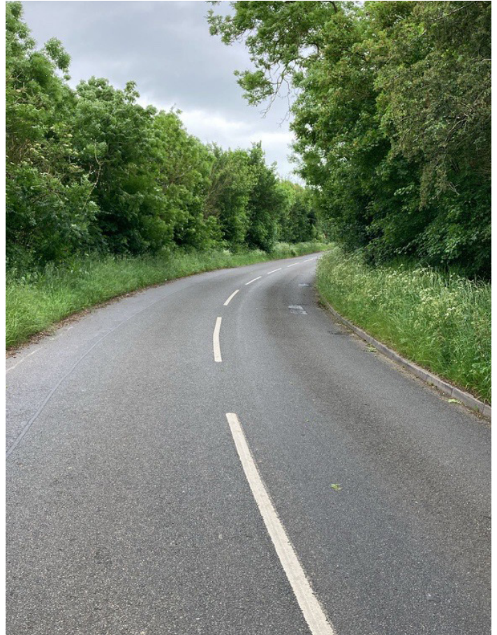
Completed reinstatement works on Little Horwood Road, May 2024
