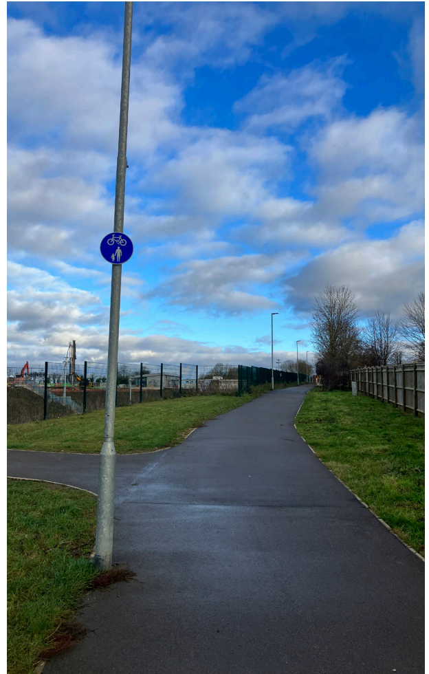
Reinstated Winslow 6/9 shared use PRoW with an upgraded cycleway
